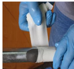
Install Plex Wrap as firm as you can
