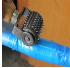
Run spike roller along Wrap
