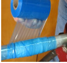
Apply constrictor Wrap
