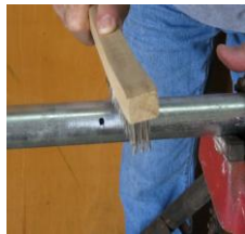
With pressure off Prep damaged area
