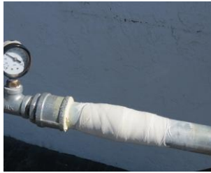
Pressure can be turned on In about 1 hour
